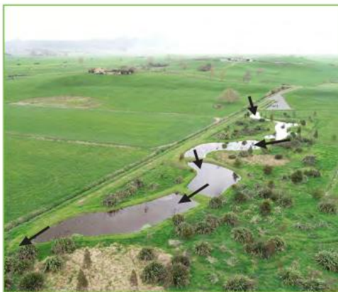
The serpentine path of the wetland excavated into a boggy area previously planted with harakeke/flax and native trees is shown soon after planting (left) and from the opposite end once wetland vegetation was fully established (right).
